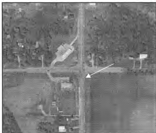
Figure 4: Aerial Image Signalized Expressway Intersection
